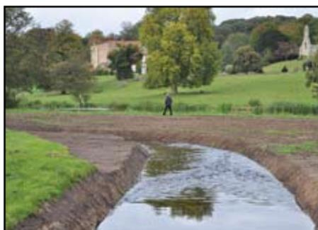
**Bayfield New River 2014.** After 120 years of being under-grounded in a brick tunnel the river alongside Bayfield Lake was brought to the surface with a new channel. The aim of the 1890's work was to avoid rapid silting up of the Lake, which had been created on the original course of the river. We now have 1.2km of sinuous new river with thirty-one riffle and pond areas. Huge volumes of soil were
